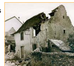
Damage observed during Arette, 1967 EQ
